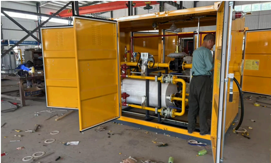
PRMS station in fabrication
